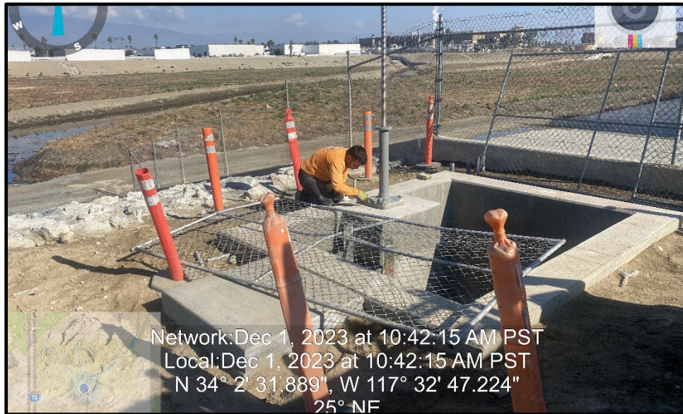
Wineville Basin Improvement – Outlet Diversion Structure (Installation of new Gate)
